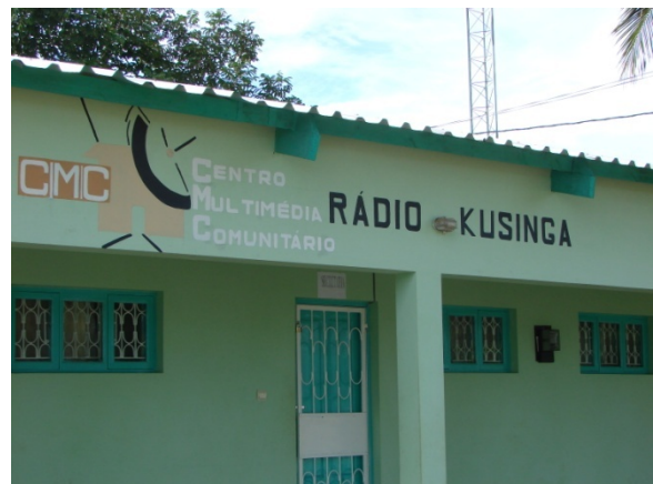
The community radio station is in Massinga. The station structure was built with contributions of the Canadian Auto Workers.
